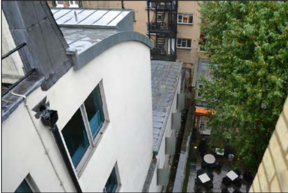
View of southern elevation of 11 Berkeley Street and relationship to the terrace at 40 Dover Street
